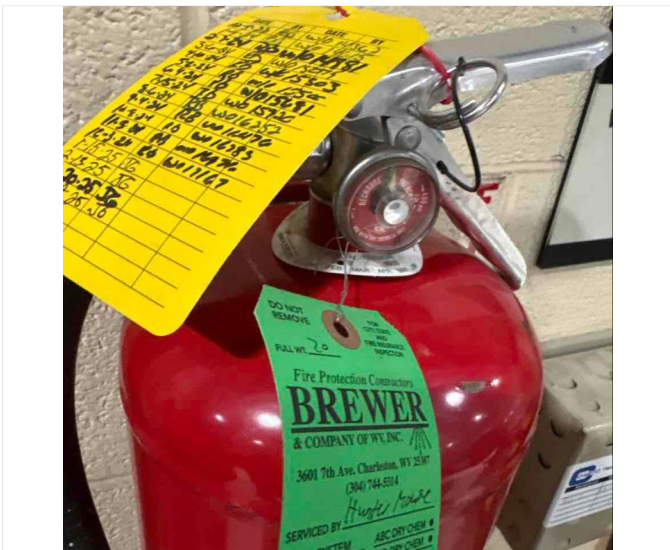
Device Type: Fire Extinguisher ScanID: NH-327320 Location: 1st motorpool 111 Work bay Service: Inspected Comment: Needs 6yr Maintenance
