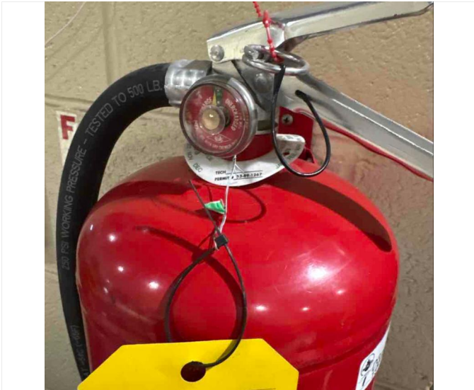
Device Type: Fire Extinguisher ScanID: NH-327319 Location: 1st motorpool 109 Workbay Service: Inspected Comment: Needs 6yr Maintenance Solution: Replace
