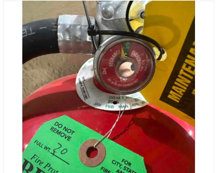
Device Type: Fire Extinguisher ScanID: NH-327312 Location: 1st motorpool 110 Workbay Service: Inspected Comment: Leak Down Solution: Replace
