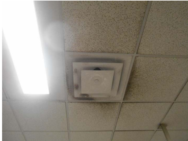
Visible Mold in the Ductwork
