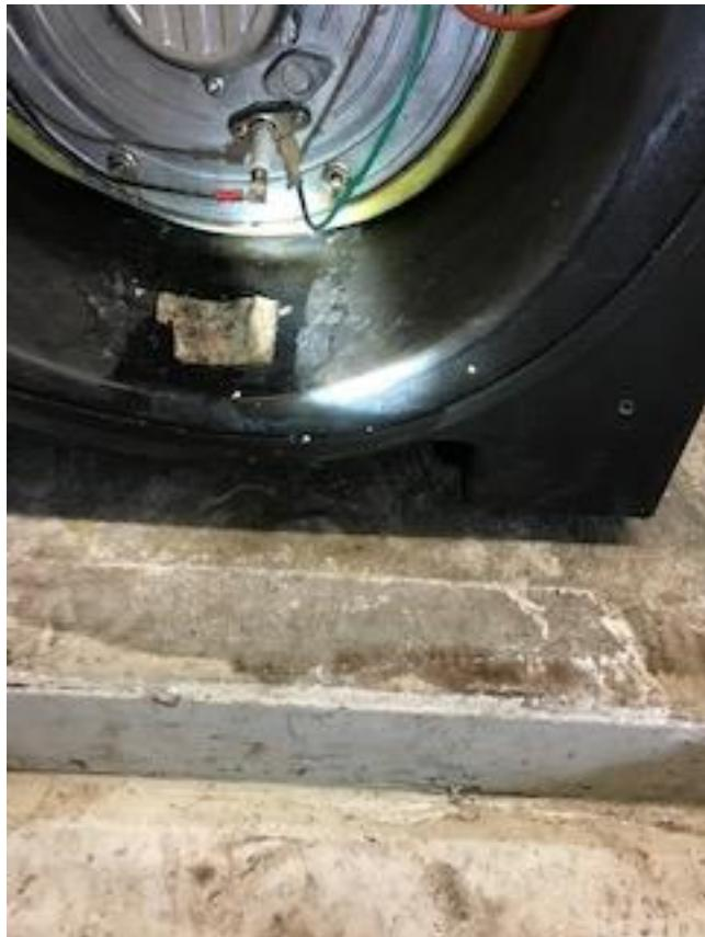
**Requirement:** The boiler is leaking in and near the firebox of this boiler. Shut down and repair or replace the boiler. In accordance with ASME NBIC.
