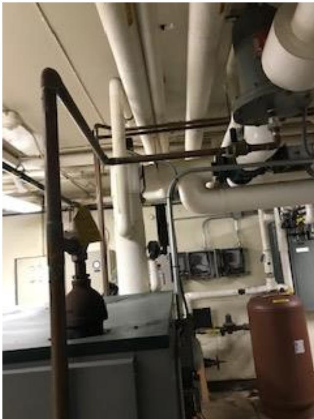
**Requirement:** The boiler relief valve should be independently piped to the drain. In accordance with Section IV.
