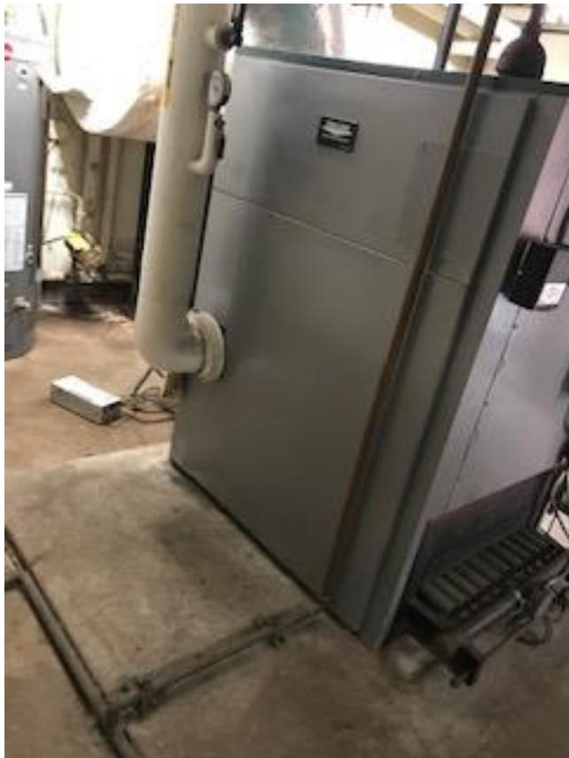
**Requirement:** Either separate the relief valve discharge piping all the way to the drain or install an increase to the piping size where it connects together. The piping shall be large enough to support the relief valve capacity. In accordance with Section IV.
