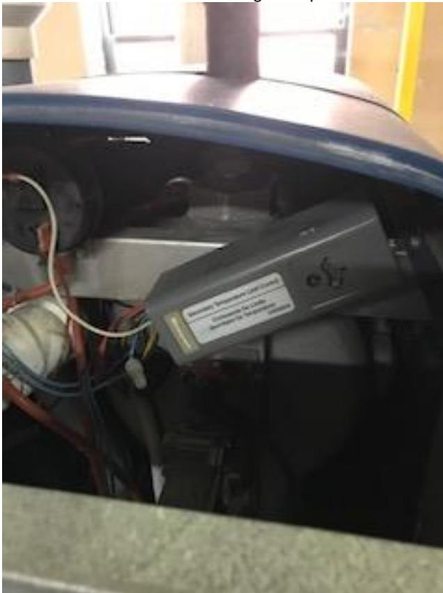
**Requirement:** Need to install a high temperature shut off with a manual reset. In accordance with ASME CSD-1.
