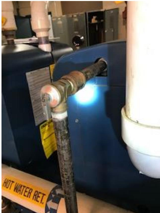
**Requirement:** Install the relief valve with the spindle in the vertical position.
