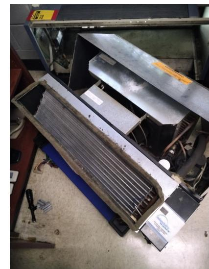
Found this ptac (Asset 4046) Room 202 in the training bldg. lock out on high pressure ,after investigating, found a piece of foam tape wedged in between the condenser and the fan schrow not allowing the fan to turn ,removed foam tape and verified operation ,p tac is running well now.
