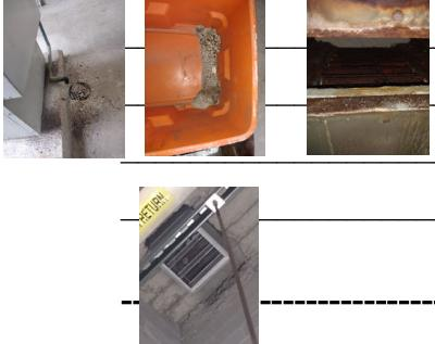
Brewer was on site and everything on their end checks out ok. Upon investigating i found the exhaust fan damper not opeing properly and the boiler heat exchanger was blocked off with rust not allowing it to properly vent the flue gases. got exhaust vent unstuck and cleaned top of heat exchanger
