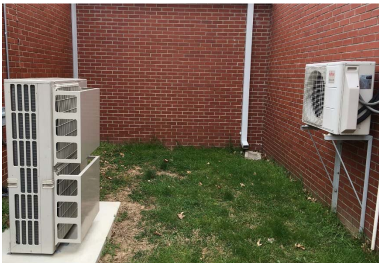
Figure 24 Ductless mini-split units
