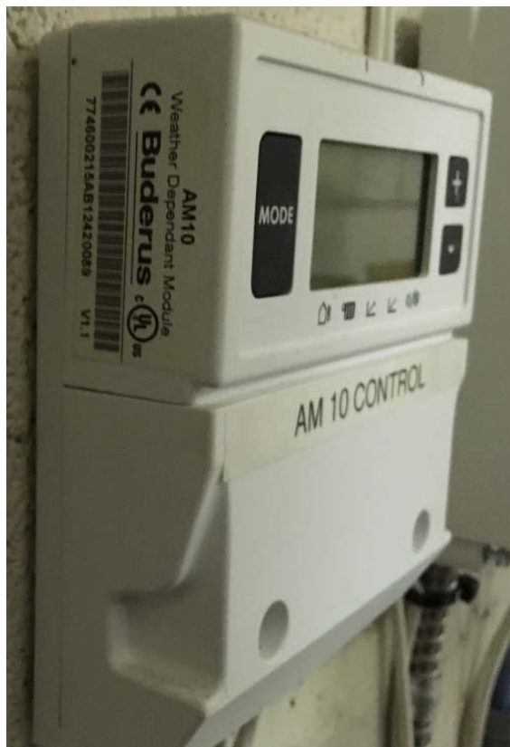
Figure 7 Buderus Boiler AM10 Weather Module
