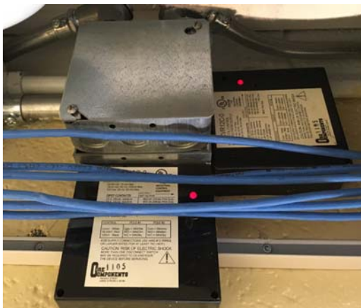
Figure 20 PTAC enable / disable and occupancy override relays
