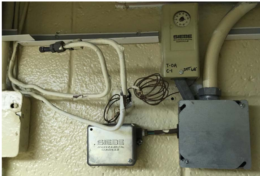
Figure 25 Pneumatic Controls
