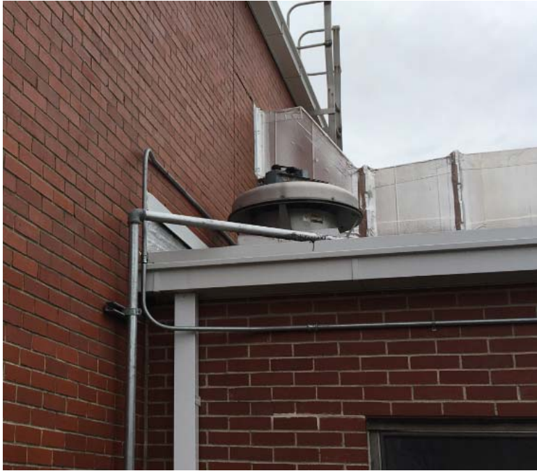
Figure 31 Kitchen exhaust fan out of service
