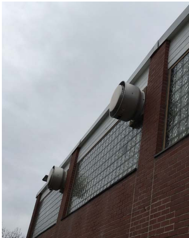
Figure 28 Exterior view of Exhaust Fans (2 of 4 shown)
