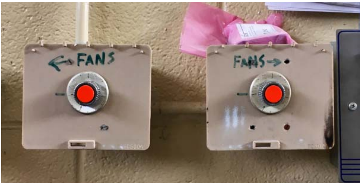
Figure 30 Exhaust fan controls
