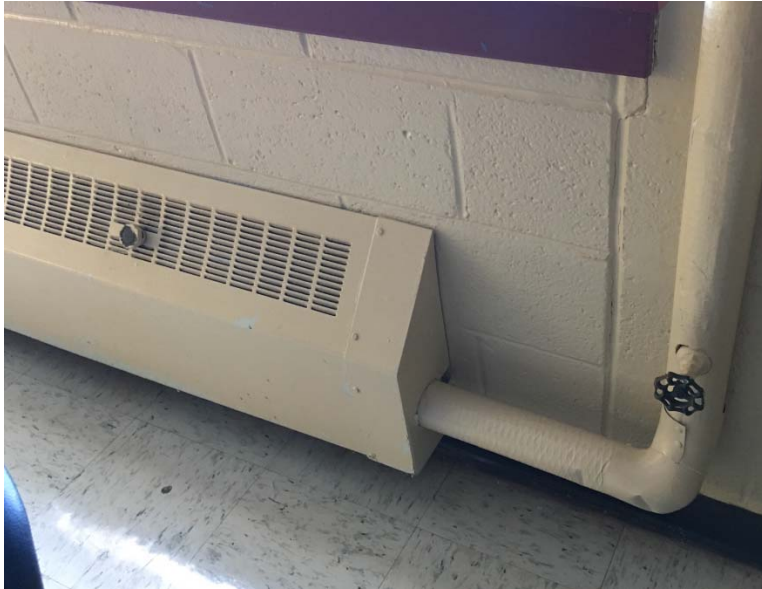
Figure 21 Hot Water Fin Tube Radiation
