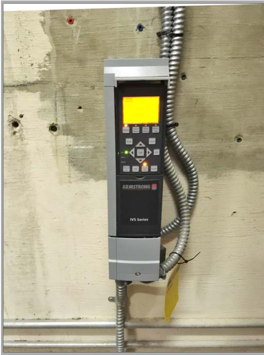
Figure 8 Pump VFD (1 of 2 onsite)
