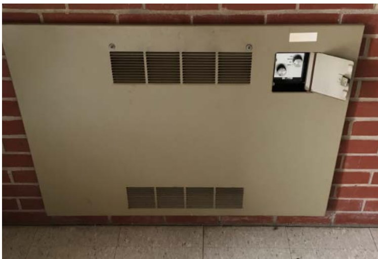
Figure 22 Hot Water Cabinet Unit Heater
