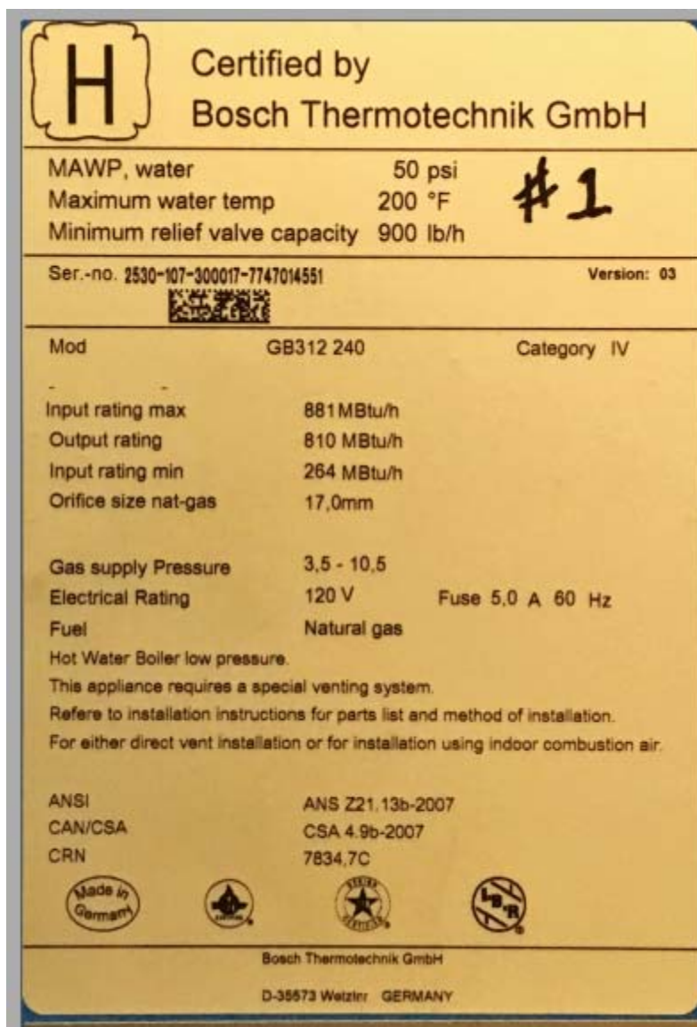
Figure 5 Boiler Nameplate (1 of 3 onsite)
