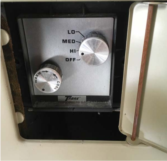
Figure 23 Hot Water Cabinet Unit Heater controls
