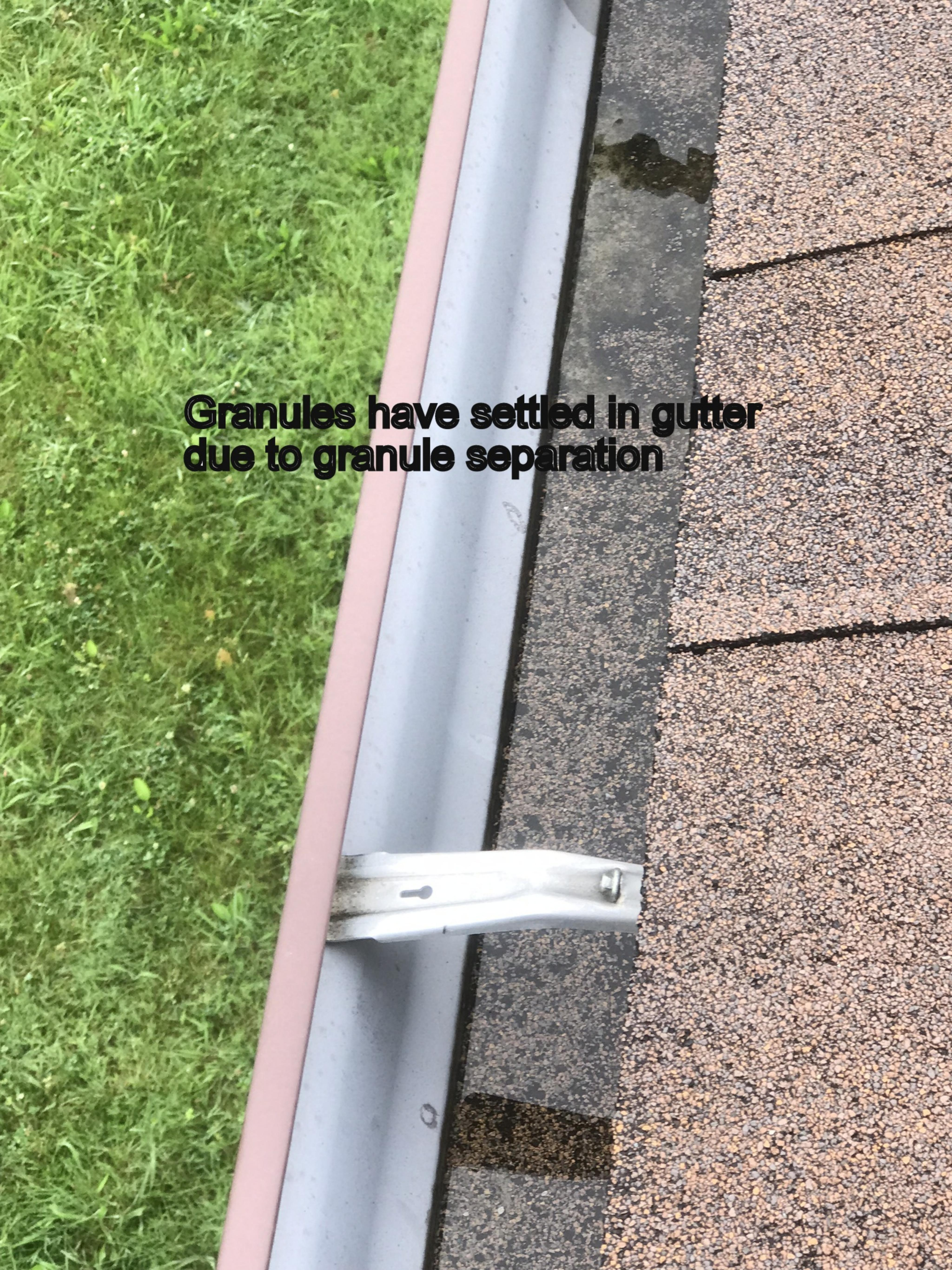
**Granules have settled in gutter
