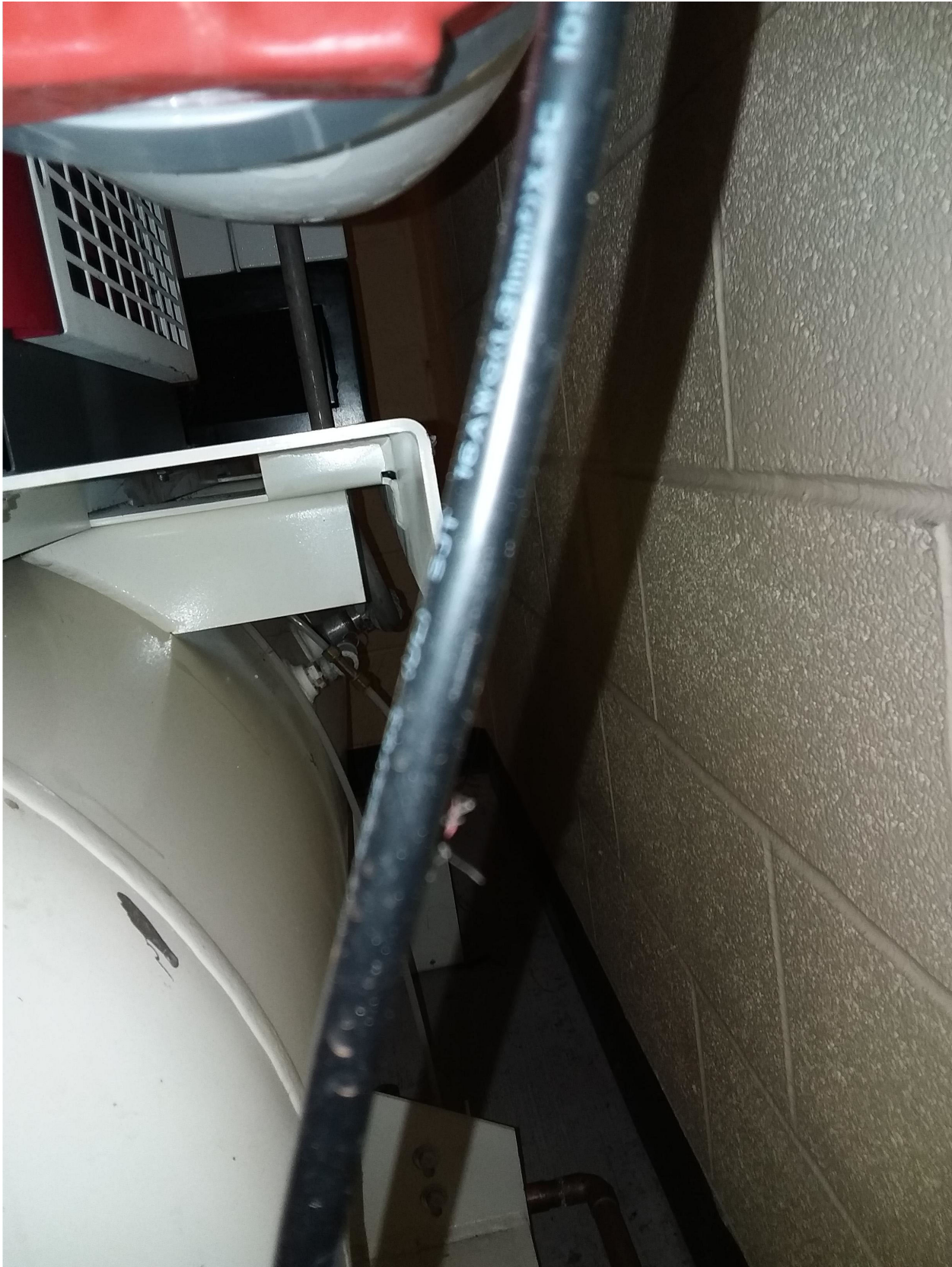
Distance between unit and sidewall 7"
