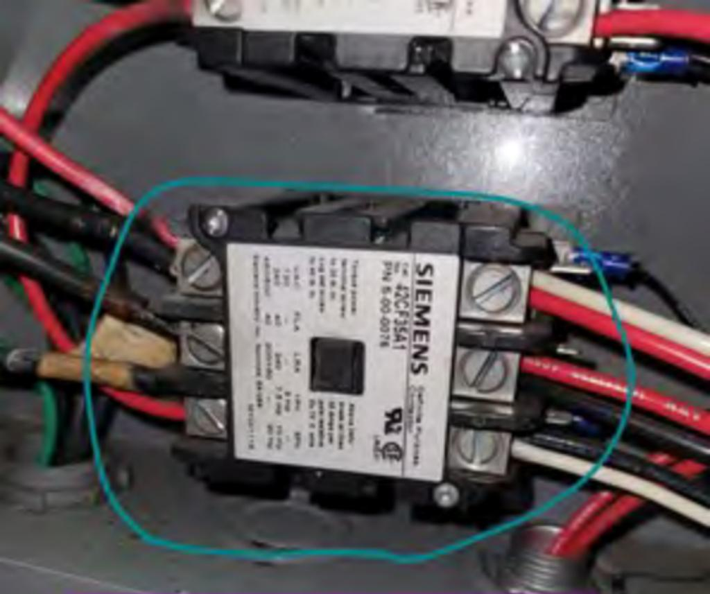
power comes in, but not out of heat coil contactor
