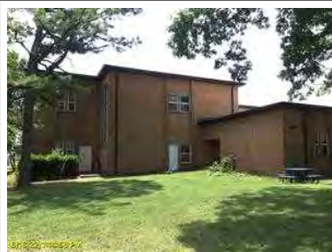
Right front section of building.
