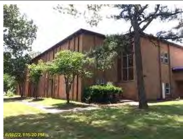
Left front corner of building.
