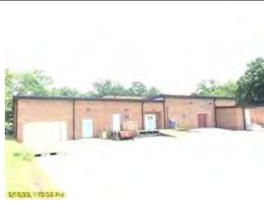
Right rear section of building.
