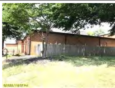
Left rear corner of building.
