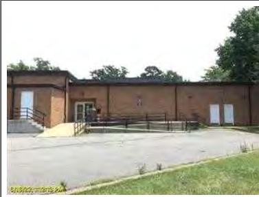
Rear main entrance to building.
