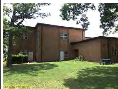
Right front section of building.
