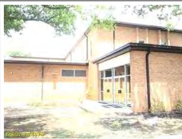
Left side section of building.
