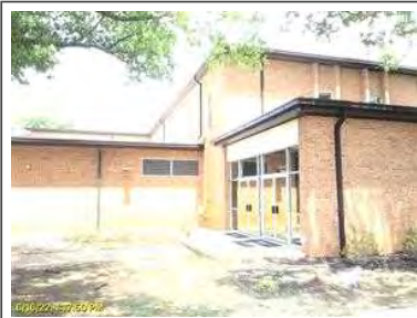
Left side section of building.
