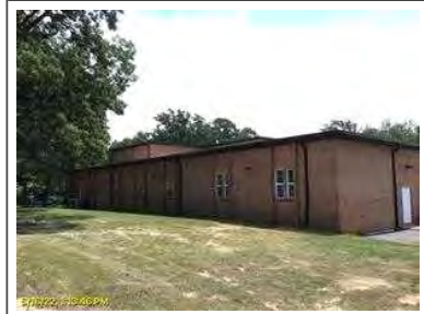
Right front corner of building.
