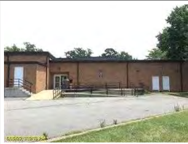
Rear main entrance to building.
