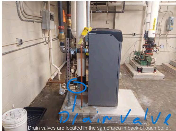
Drain valves are located in the same area in back of each boiler.
