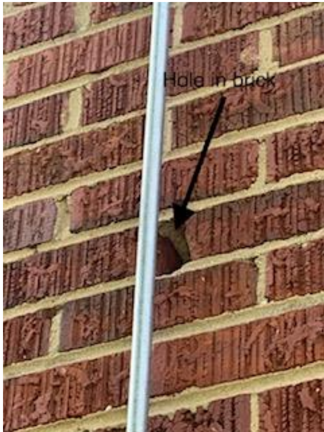
Hole in front wall near camera of training building MD021
