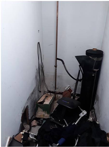
(cm) - Sump pump is not plugged in and area is heavily obstructed with random items
