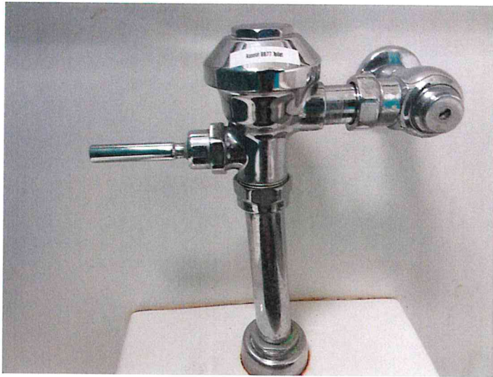
old flush valve and vacuum breaker
