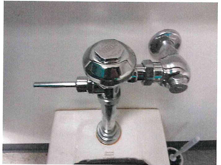
new flush valve and vacuum breaker
