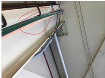
**P55.1:** Recommend replacing the bent bar
