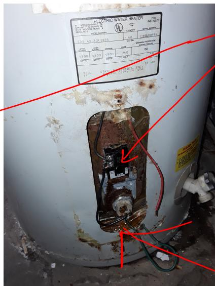
Replaced upper and lower thermostats and amped heaters.
