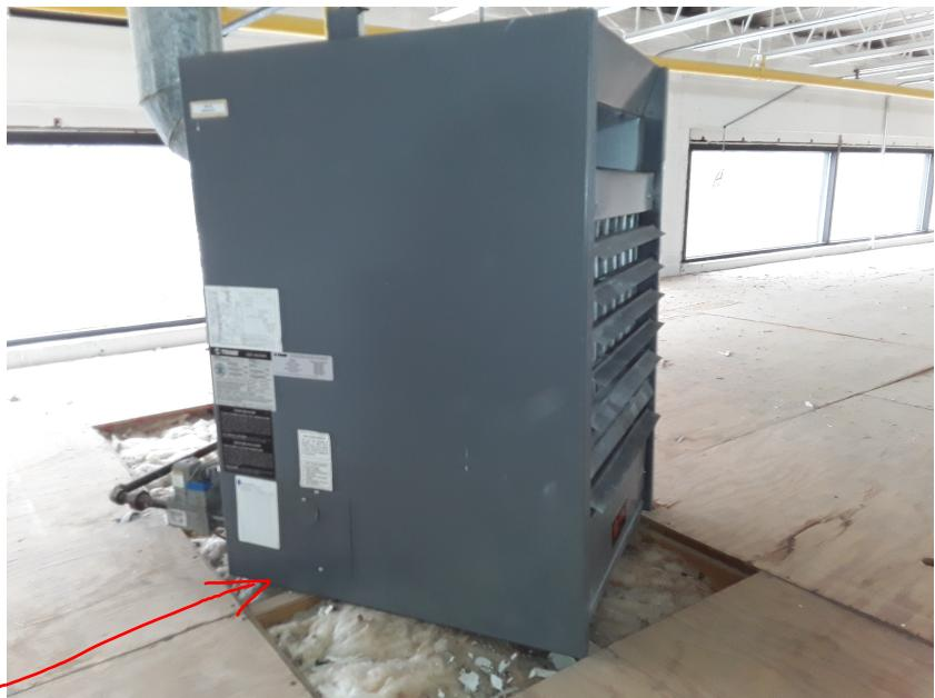
Suspended gas heater is to close to wood!
