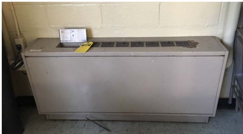
Figure 13 Older model PTAC (TPI Corporation RM135A-W)
