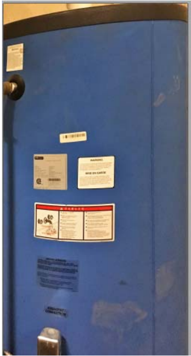
Figure 9 Bosch Domestic Hot Water Heat Exchanger / Storage Tank
