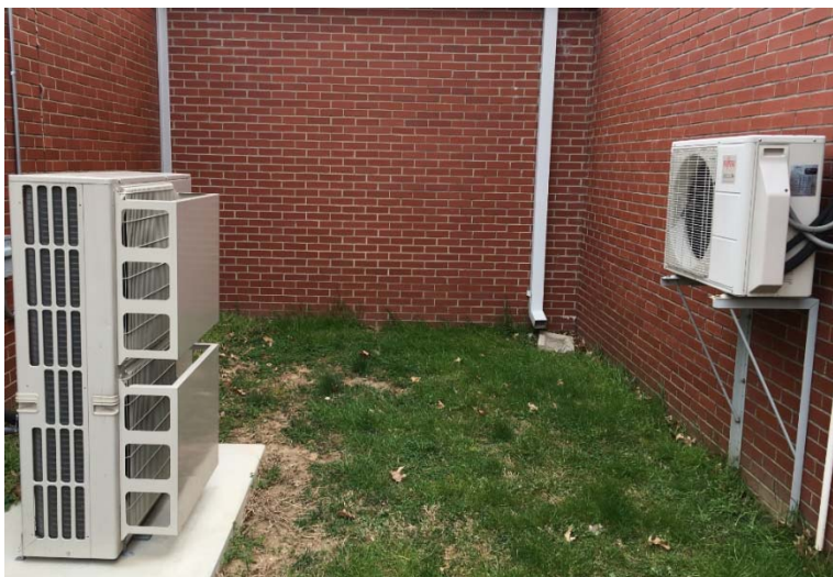
Figure 24 Ductless mini-split units
