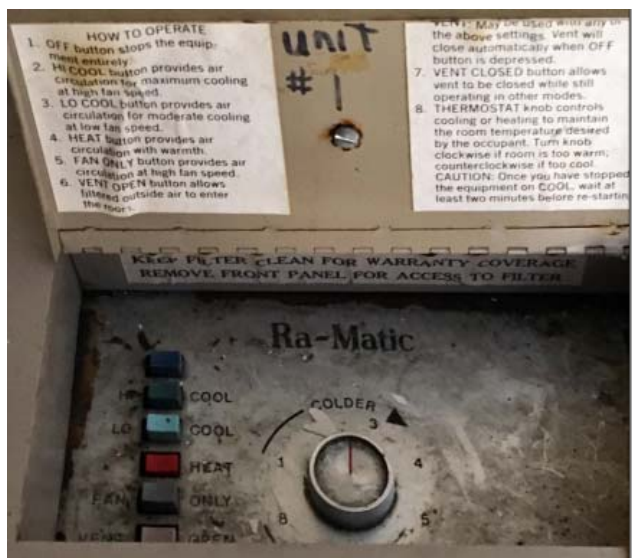
Figure 14 Older model PTAC local controls
