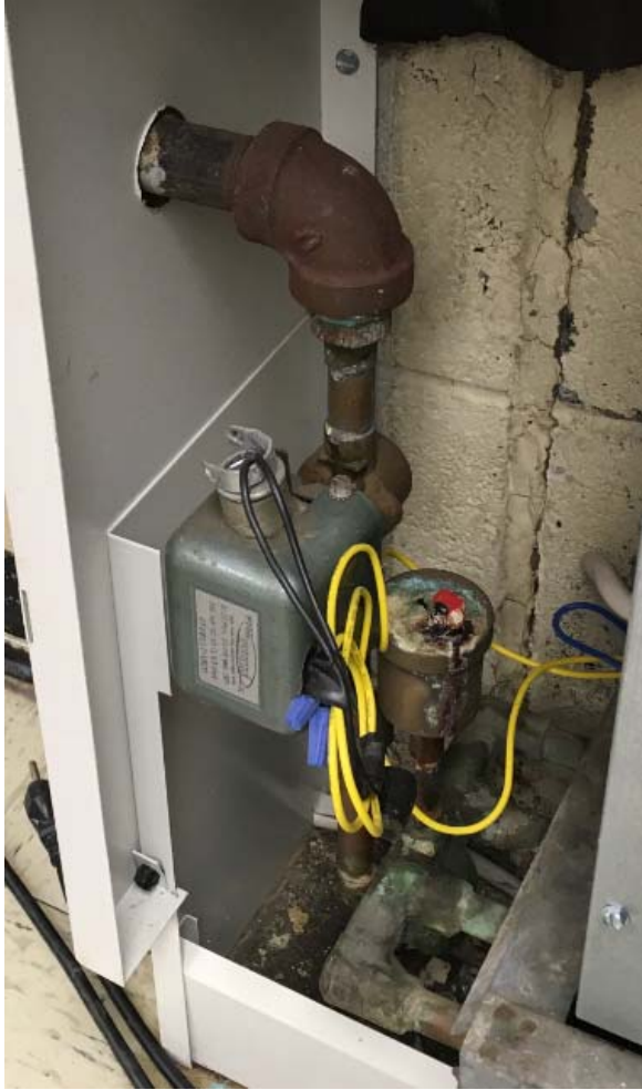
Figure 19 PTAC 2 position (non-modulating) control valve
