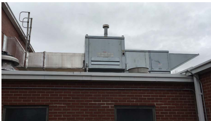
Figure 26 AHU-1 (Rupp Model R2-IBT-300-G15)
