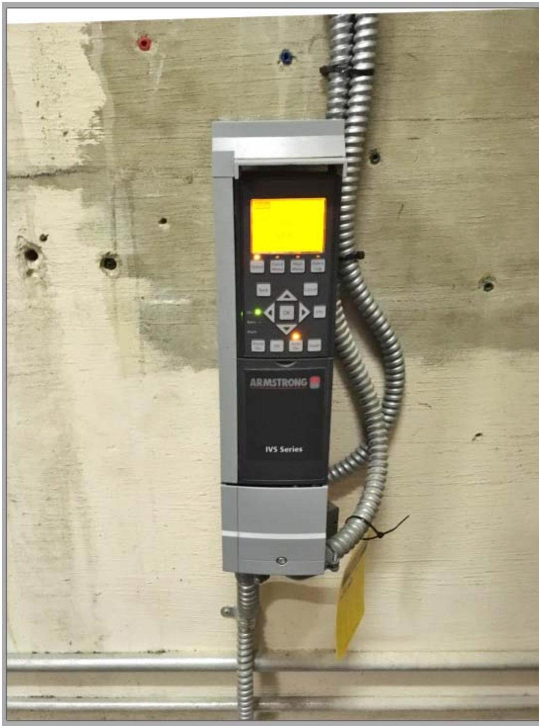
Figure 8 Pump VFD (1 of 2 onsite)
