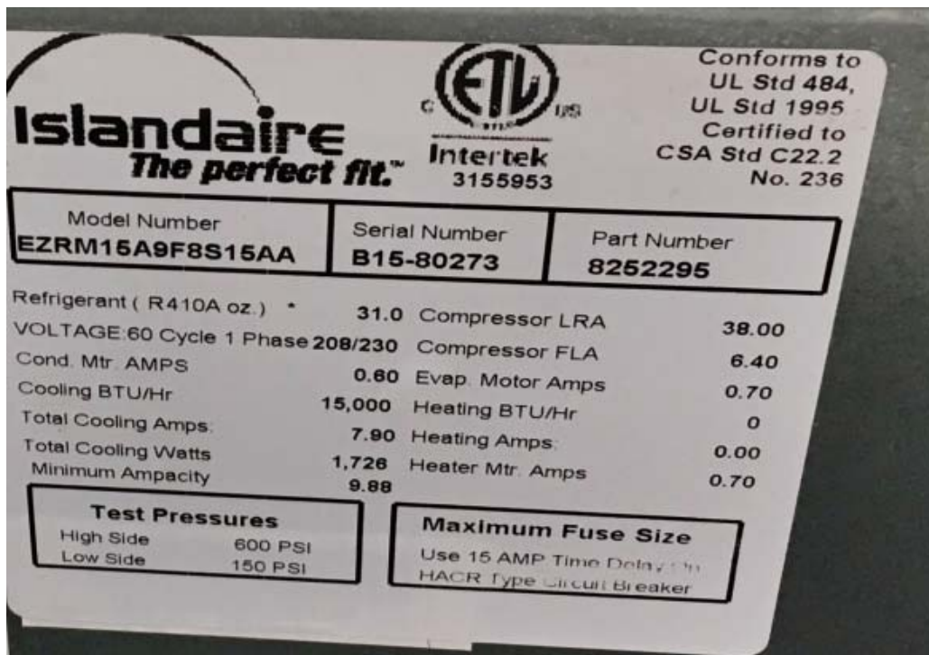
Figure 18 Newer model PTAC nameplate
