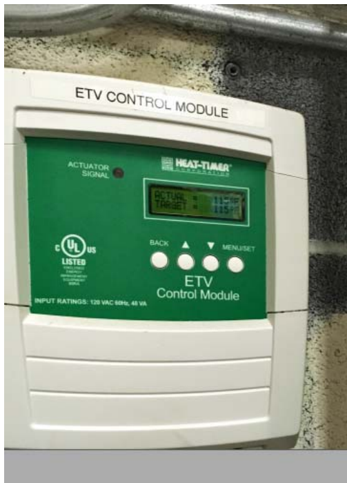
Figure 10 Heat-Timer ETV Control Module
