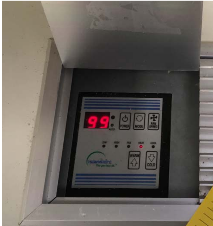
Figure 17 Newer model PTAC controls
