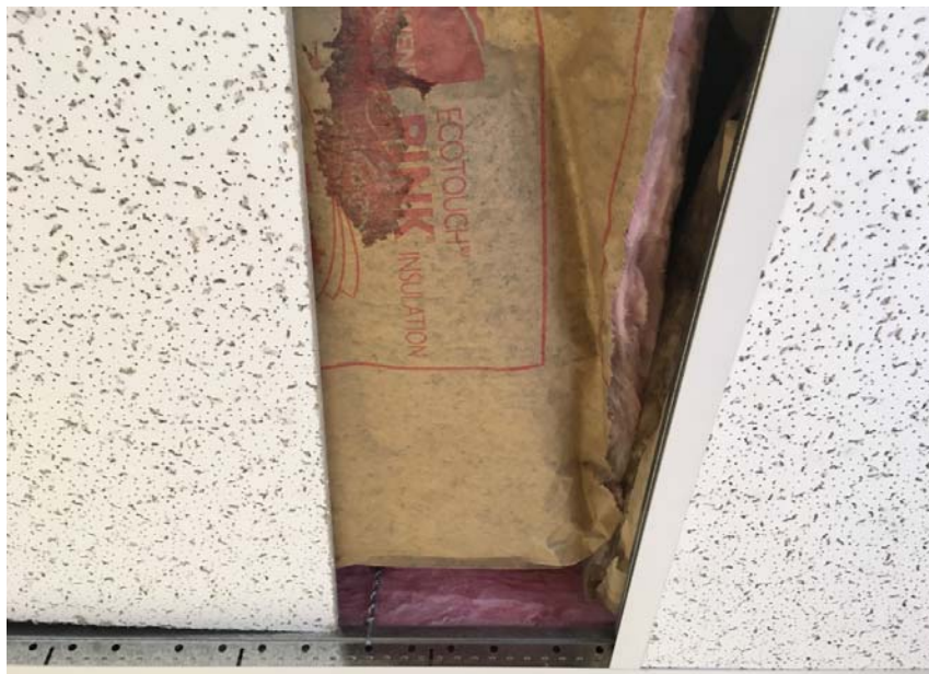
Figure 36 Low ceilings and fiberglass insulation will make for difficult wiring install
