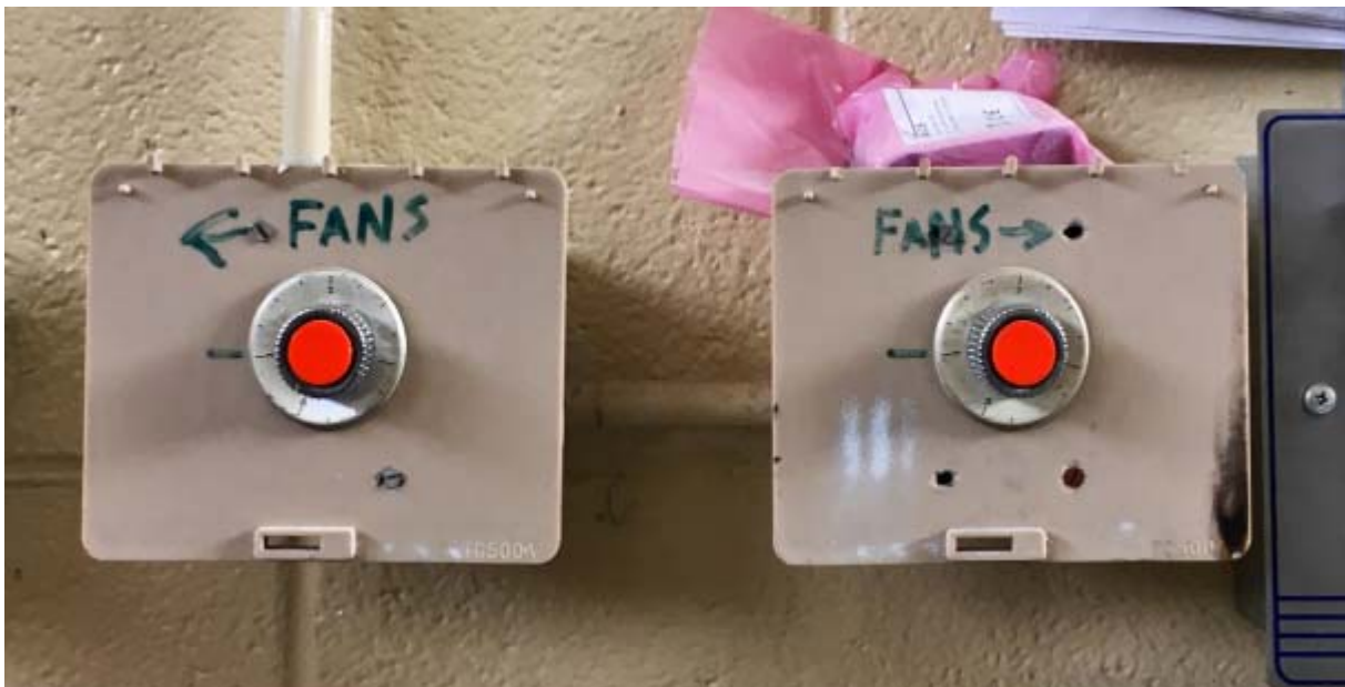
Figure 30 Exhaust fan controls
