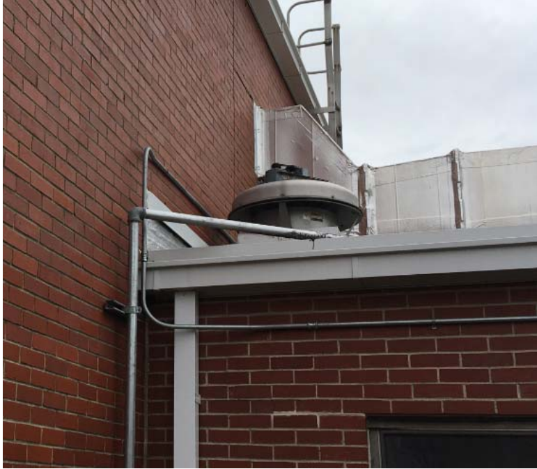
Figure 31 Kitchen exhaust fan out of service
