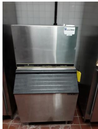
The ice machine does not operate. Checked ice maker has bad compressor. Jennifer is aware that the ice maker is not in operation.
