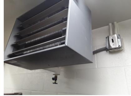
Unit in Assembly Hall shows signs of leakage and corrosion
