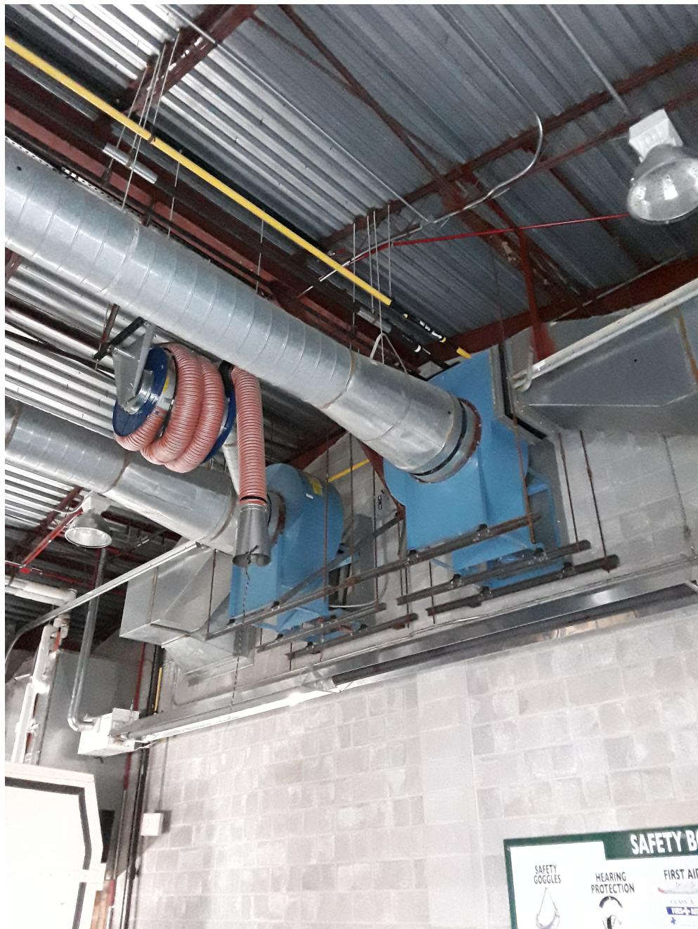
Wash bay fan has failed transformer and not working.
