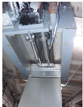
Asset #4283 - 2nd Bay heater has cracked heat exchanger. I turned off switch on heater and tagged - Danger
