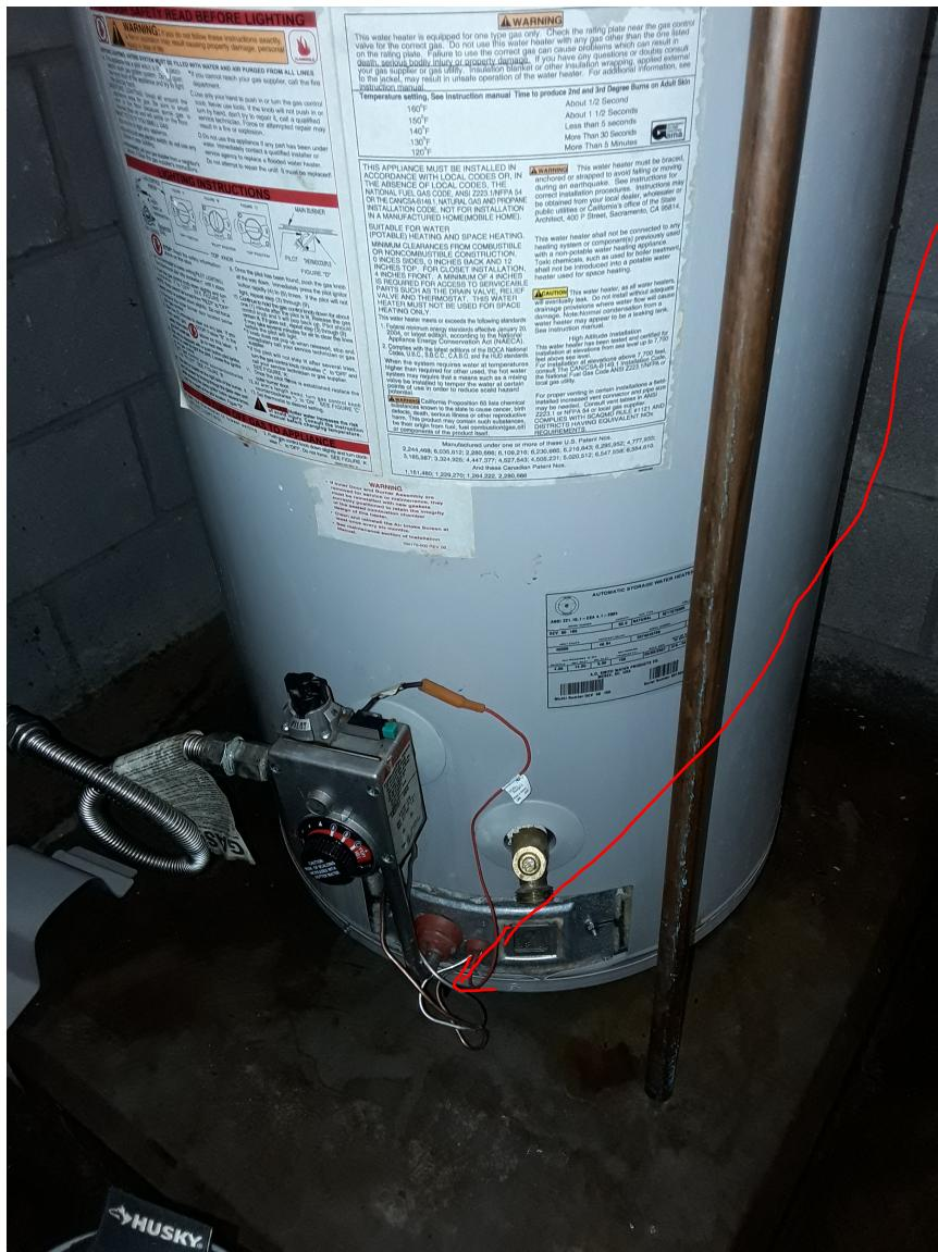
Replaced pilot assembly and pop-off valve. Working properly
