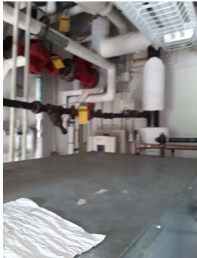
Note: Pumps in main building do not operate due to no domestic water to building.
