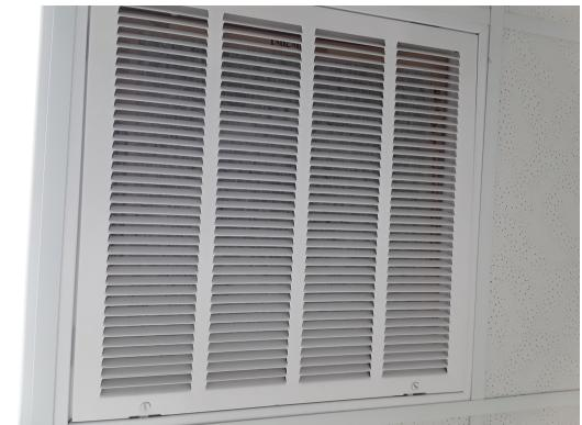
Note: none of the filters on the site are dirty. Hvac is not in operation due to faulty refrigerant lines being ran throughout the building causing multiple refrigerant leaks. AFOS is aware of these issues.
