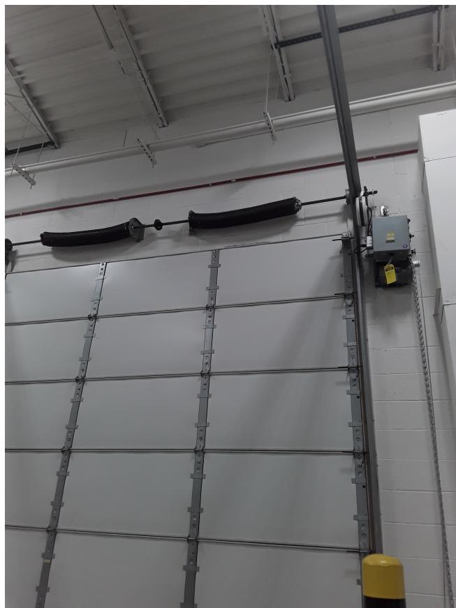
Asset # 7844 - Replaced belts on 3 operators. Belt size for all 4 operators: 5L 280.
