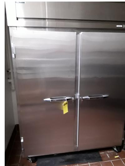
Note: Both freezers on site do not operate. compressors are bad on both. AFOS is aware both freezers are not in operation.
