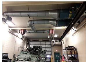
\* Ductwork loose from Unit in Washbay.
