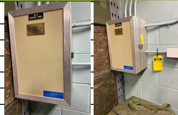
Because pallets are stacked so close to the panel the door cannot be opened.
